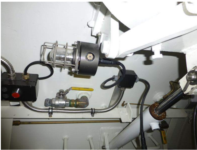
11. 6 x junction boxes and wiring
