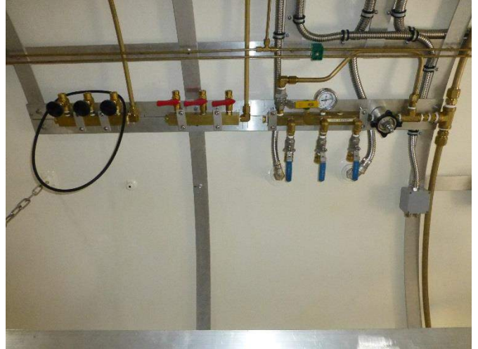
18. O2 injection pipework and valves
