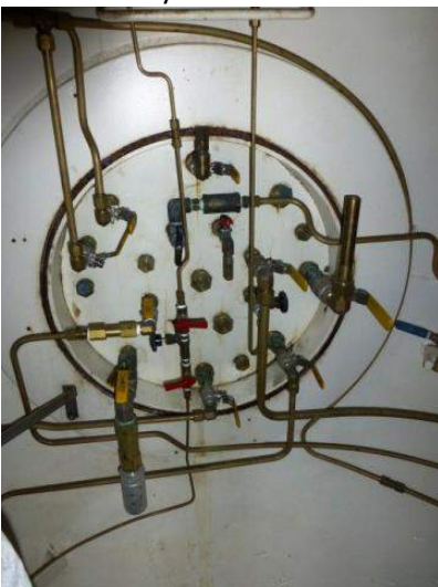
7. All pressurisation, exhaust pipework, depth and analysers
