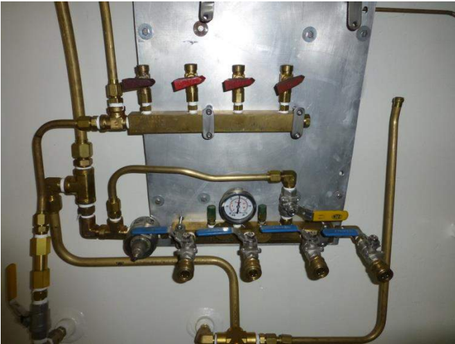
5. 2 x incomplete oxygen BIB manifolds
