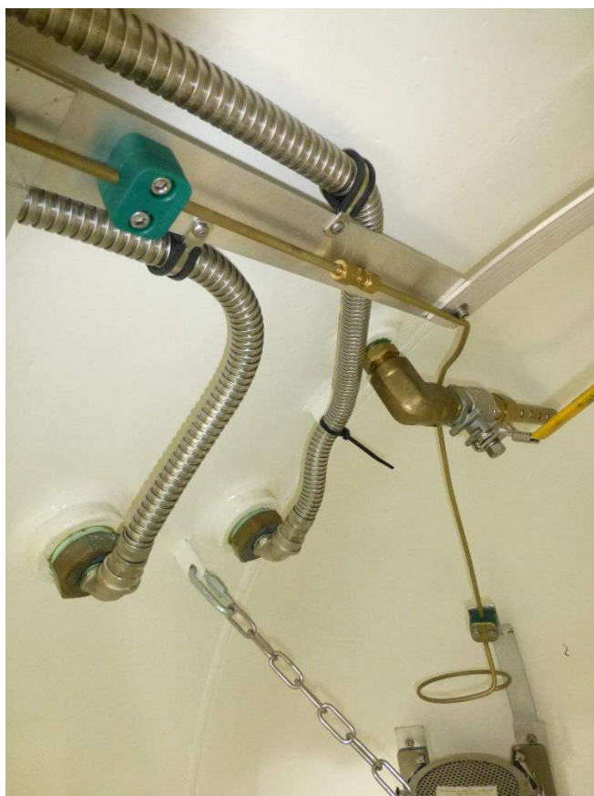
4 x electrical multiway penetrators (cont)
