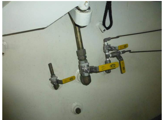
15. BIBs quick connects and 1st stages
