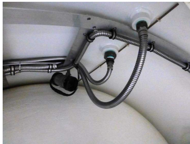
17. 4 x electrical multiway penetrators fitted 3 M/L, 1 E/L
