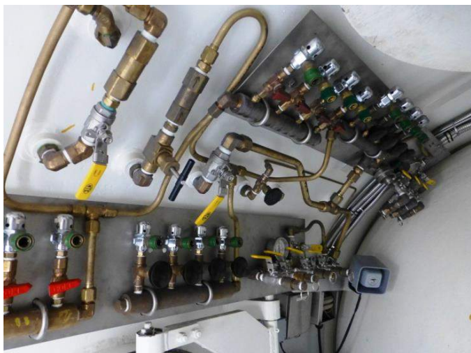
7. 1 x 8 way mixed gas BIBs manifold
