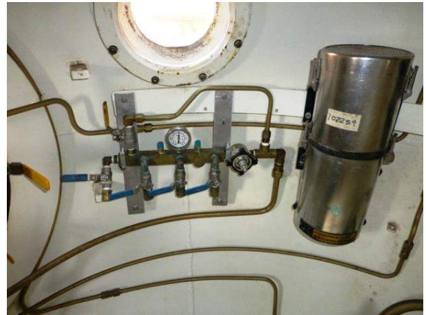
8. Oxygen injection lines pipework and valves
