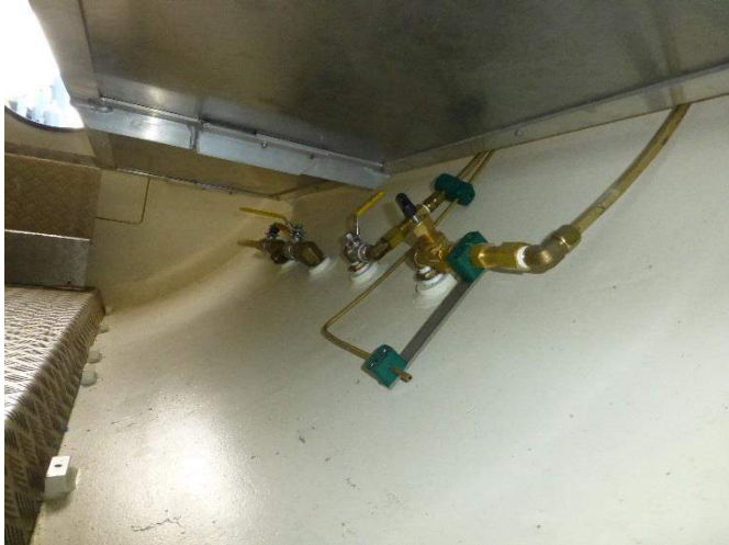
17. 1 x 3 way mixed gas BIBs manifold
