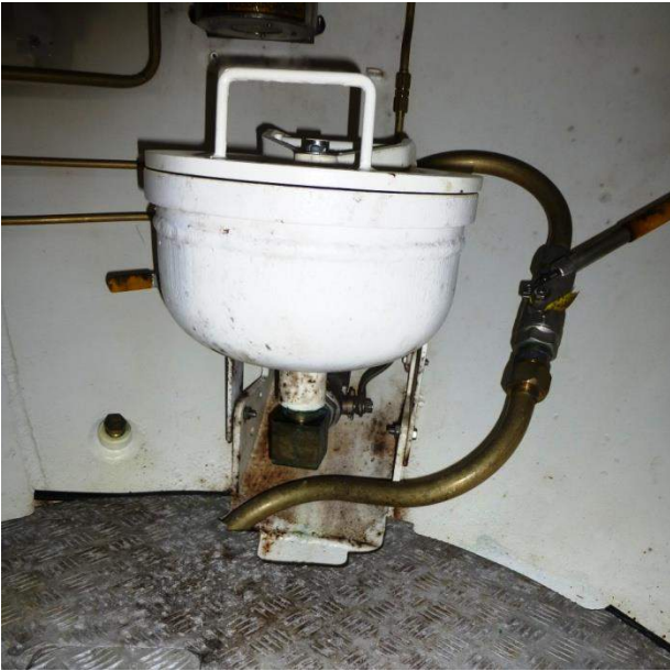
5. BIBS manifold oxygen x 4
