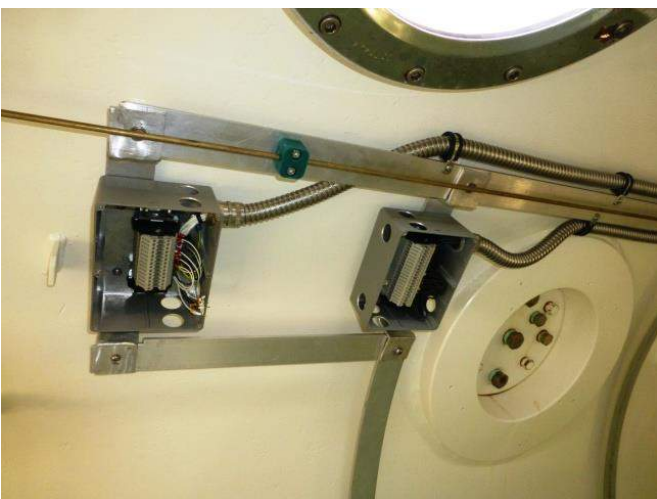
6. 4 x electrical junction boxes with wiring to electrical penetrators
