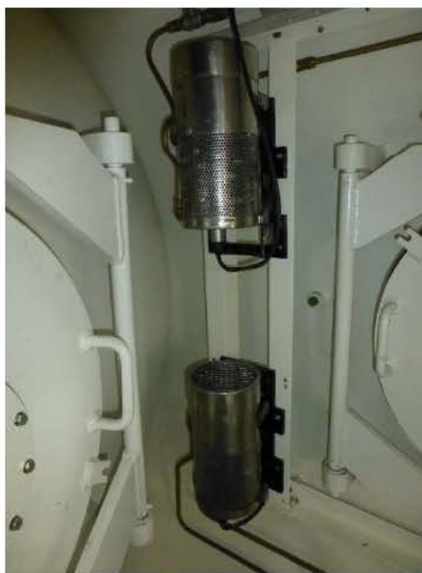
12. Exhaust BIBs and manifold and pipework and BPR
